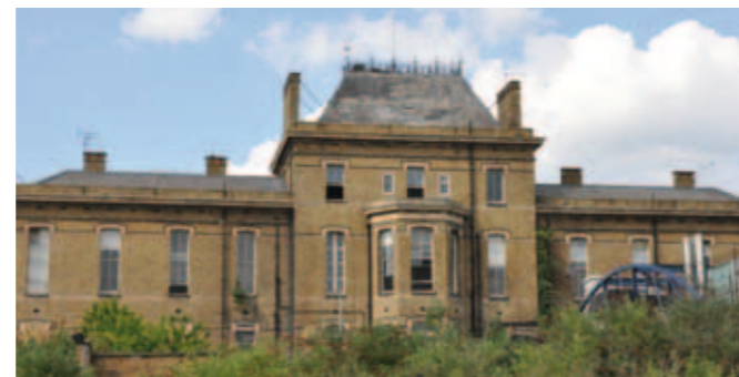
Above: The derelict hospital acquired by Berkeley
