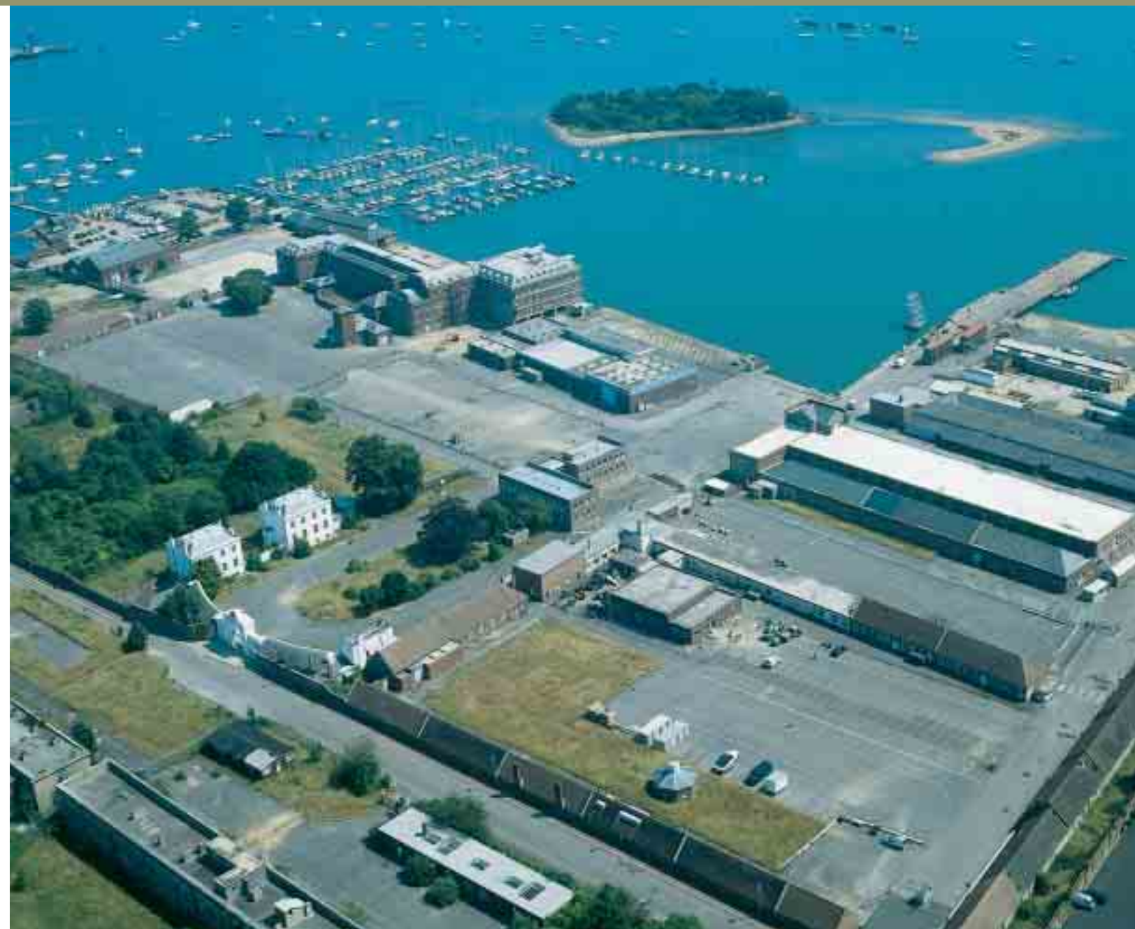
At Royal Clarence Yard, Gosport, Berkeley Homes conducted a series of community planning events, allowing it to work up its development plans for the refurbishment and regeneration of the former naval yard in partnership with local people.
