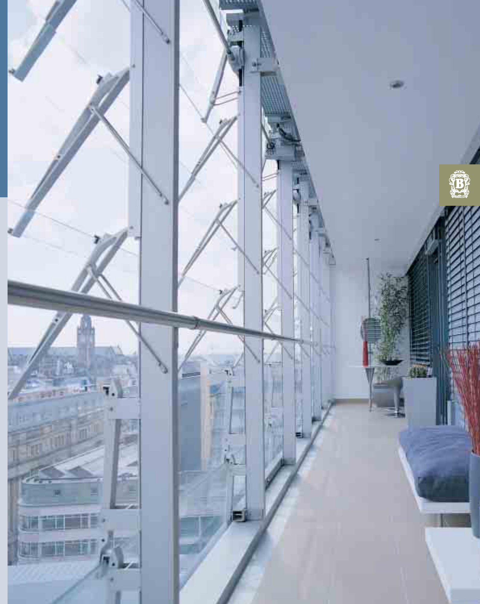
The automated louvres at No. 1 Deansgate, Manchester, assist with the natural ventilation of the building and provide a 'buffer zone' between the exterior and main living areas of the development.
