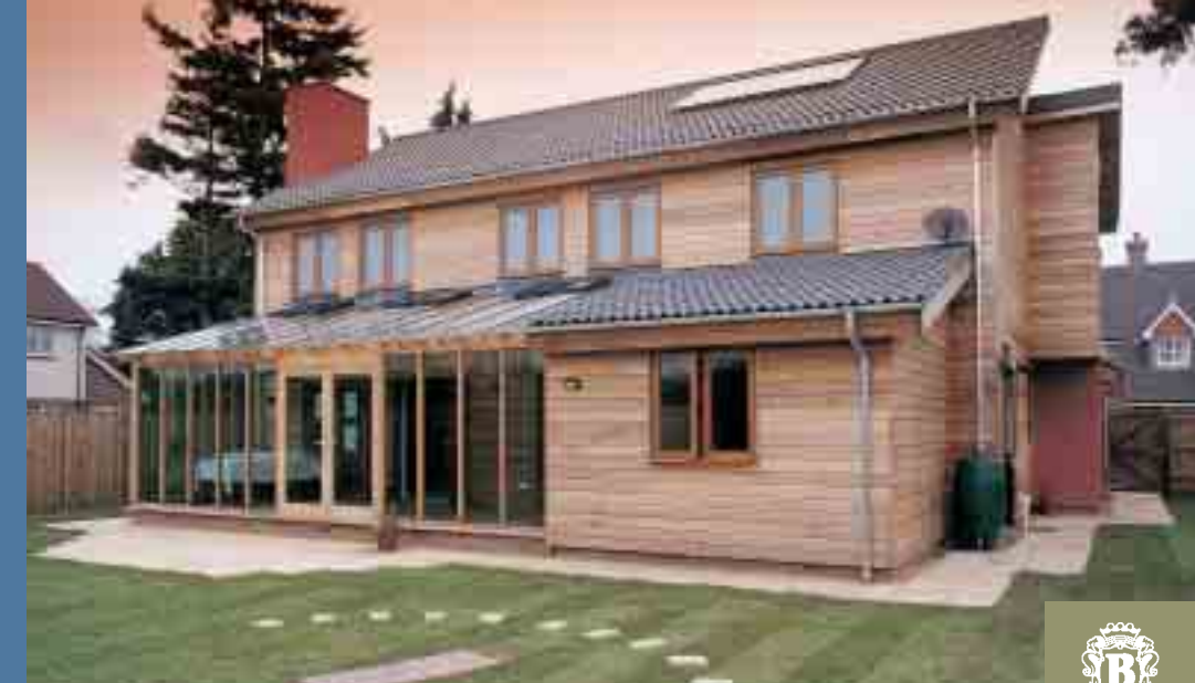
Integer House in Newbury is a prototype development project for open market sale that is truly energy efficient.
