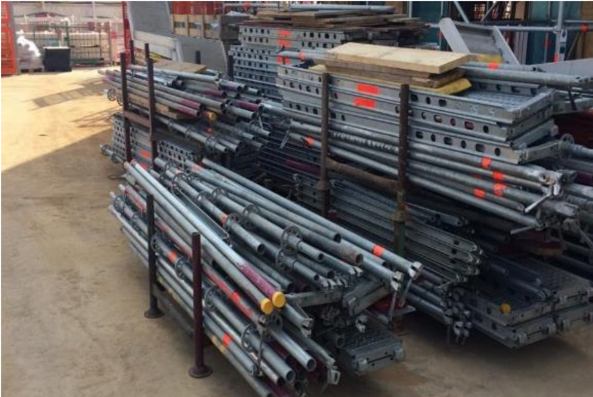
All scaffold tubes and lengthy components shall be stored in proprietary stillages.
