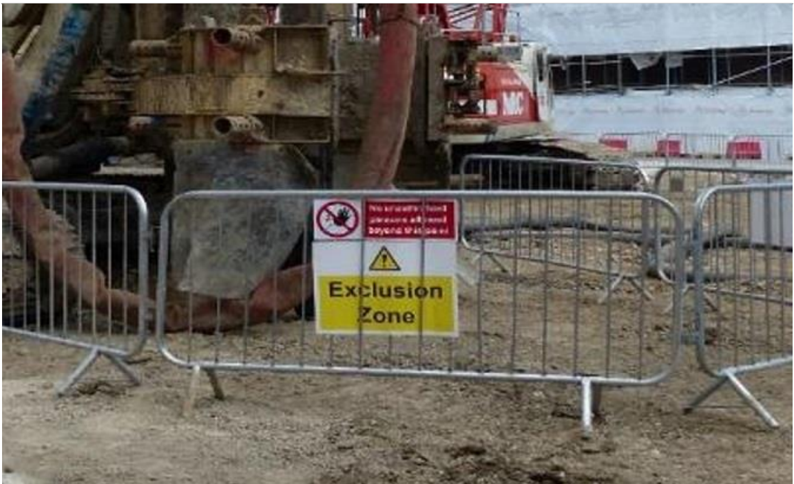
All work areas that restrict access shall be sufficiently protected by physical measures, such as proprietary barriers or tube and fitting scaffold, and shall prominently display signage detailing the access restrictions.
