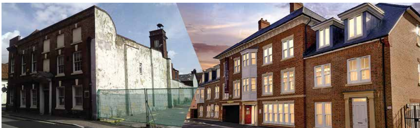
Churchill Living's Sarum Lodge – a new retirement community, located on a previously derelict, town centre, brownfield site in Salisbury - before and after.
