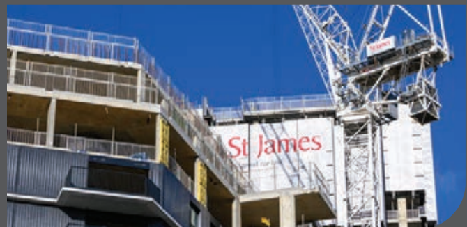
Construction activities at White City Living
