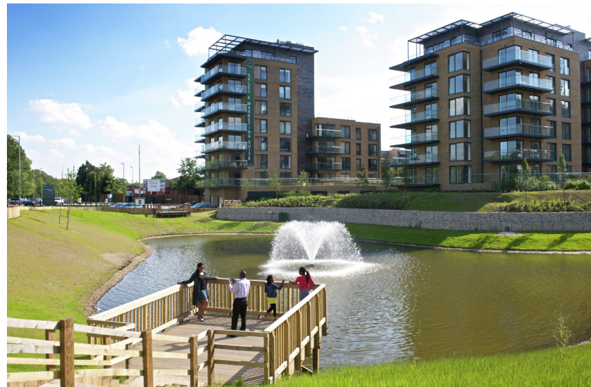
Flood attenuation pond at Kidbrooke Village
