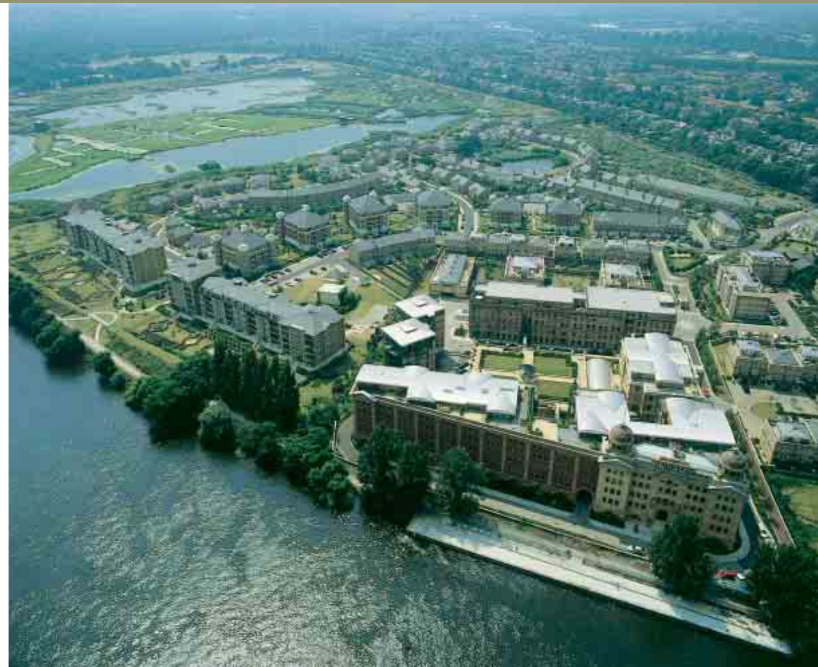
An aerial view of Barnes Waterside and the Wildfowl and Wetlands Trust, where part of the development included converting 4 concrete reservoirs into more than 30 different habitats. This site was the Global Winner of the British Airways Tourism for Tomorrow Awards 2001.
