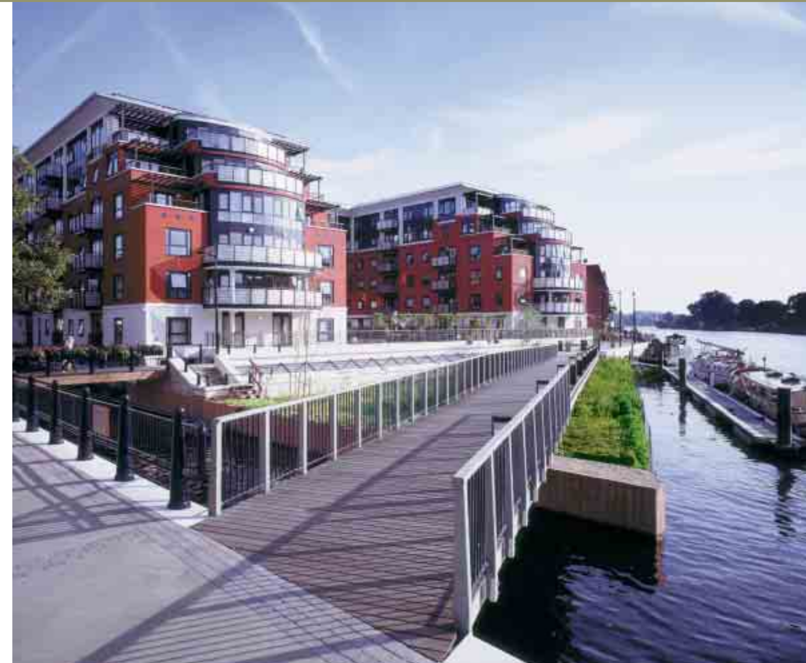
Charter Quay, a mixed-use scheme in Kingston upon Thames which, through consultation with the local community and relevant authorities, will deliver a 1,100 seat theatre, new moorings and a walkway past the wetlands, as well as other local leisure amenities.
