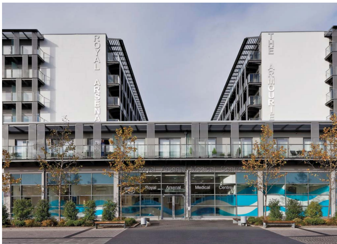
The medical centre at Royal Arsenal Riverside
